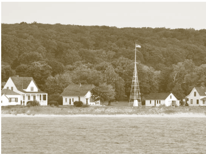
North Manitou Island. Photo courtesy of Meggen Watt, 2010
